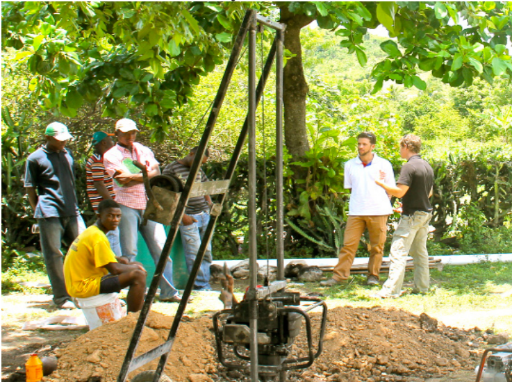
Drilling under way.
